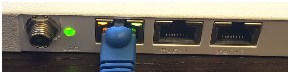
Figure 12: The SensArray has finished booting and is ready for operation.
